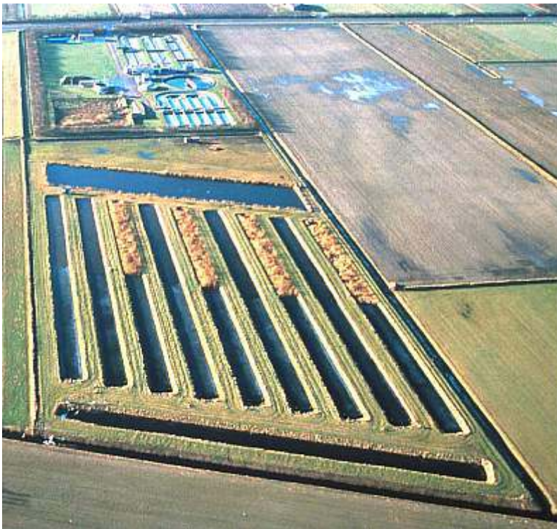
Figure 8-68: Polishing constructed wetland Eversteekoog, Texel, The Netherlands (IEES, 2013).
