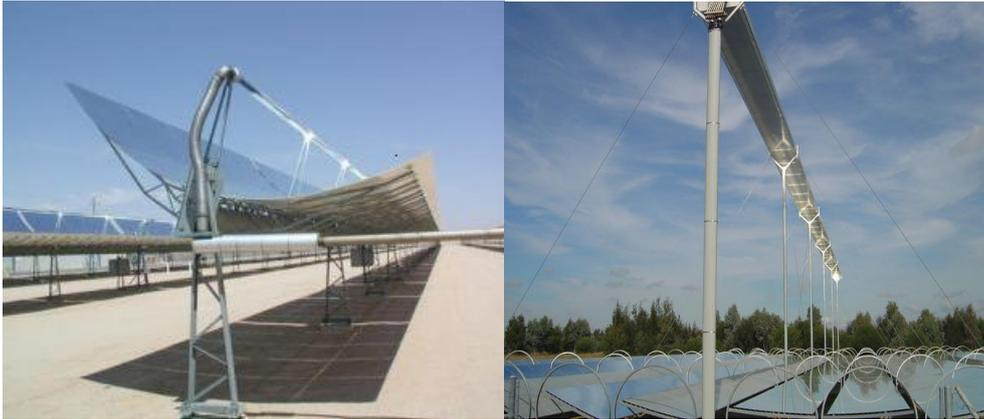
Figure 3.6 - Parabolic Trough and Compact Linear Fresnel collectors
