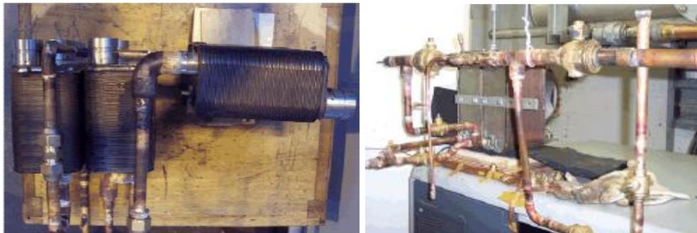
*Figure 6.6 - Evaporator (Left) and Condenser (right)*
