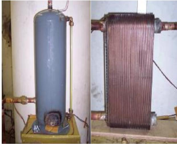
Figure 6.9 - Liquid receiver and subcooler
